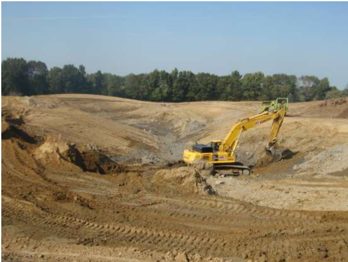
Pond Construction at the 11 th hole
