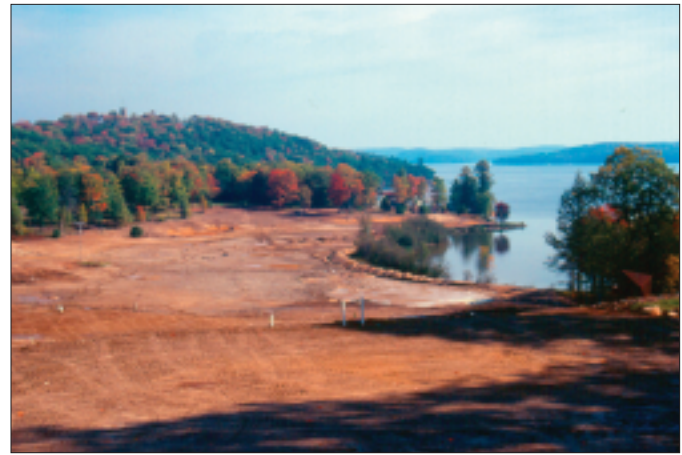
Bigwin Island Golf Club, Huntsville, Ontario. 18 th hole construction.
