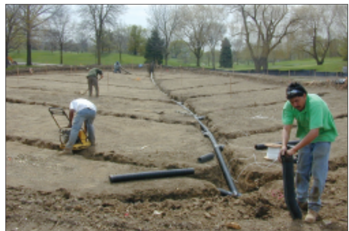
Practice tee drainage installation.
