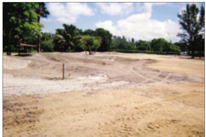
Riviera Country Club under renovation.
