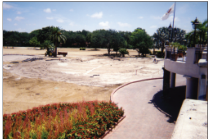
Riviera Country Club under renovation.
