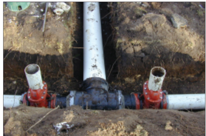
Irrigation and fitting installation.
