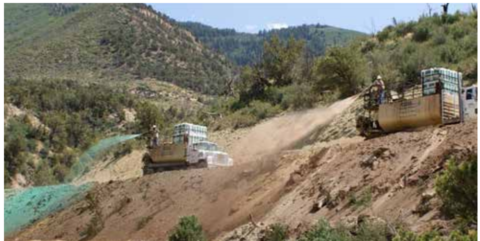
On these challenging sites, ProGanics is applied to depleted soils and then covered with Flexterra FGM to stabilize slopes and maximize erosion control
