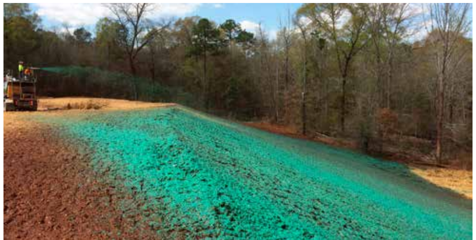
High quality grass development can be accelerated on depleted soils, by applying growing media through a hydroseeding machine
