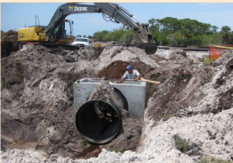
Pipe drainage was installed to carry flow off runways and under the course
